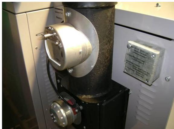
Fit the chimney starter flue to the smoke box using the screws and gasket
