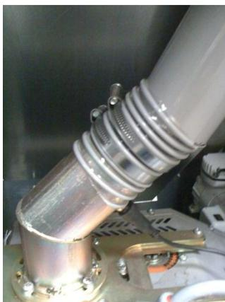
Fit flexi-pipe and hose clamps securely
